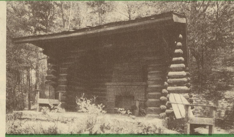
TRAIL SIDE SHELTER—CANTWELL CLIFFS
